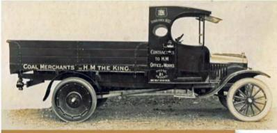
The truck used by the Coal Merchants to His Majesty the King had a dump body fitted with steel-disc wheels with solid rubber tires at the rear. The Ford TT had a one-ton rating, but we're sure more was loaded into the bed.
