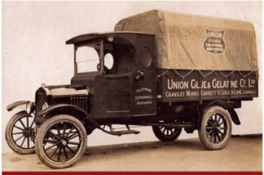
Large, curved wooden hoops that rose up from the sides of the body would be used to support a canvas tarp that was then tied down with rope, making its removal easy.
