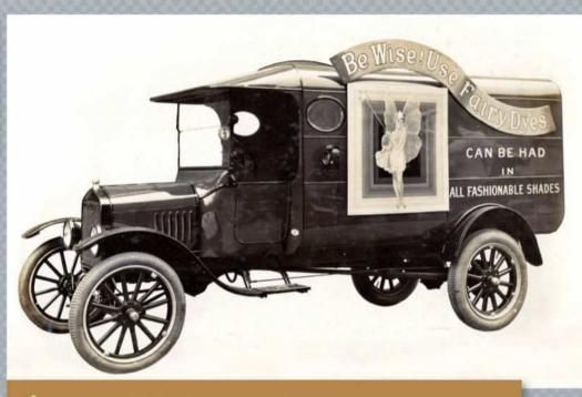
This body on a one-ton Model TT truck chassis has an elaborate ribbon-shaped sign and a huge painting of a fairy that was the logo for the Fairy Dyes company that bought the truck. Sidelamps were fitted below each oval window.
